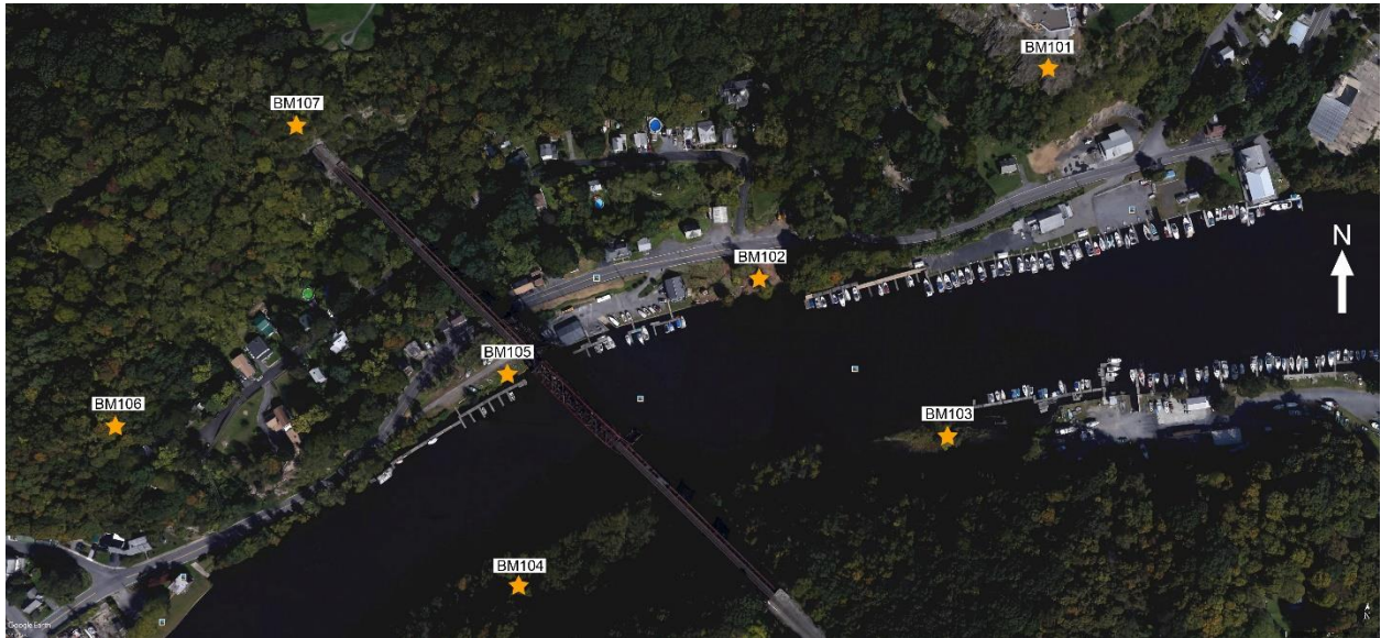
FIGURE 1. Google Earth plan view of CSX Wilbur Bridge showing instrument locations.
